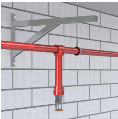
Installation de sprinklers
